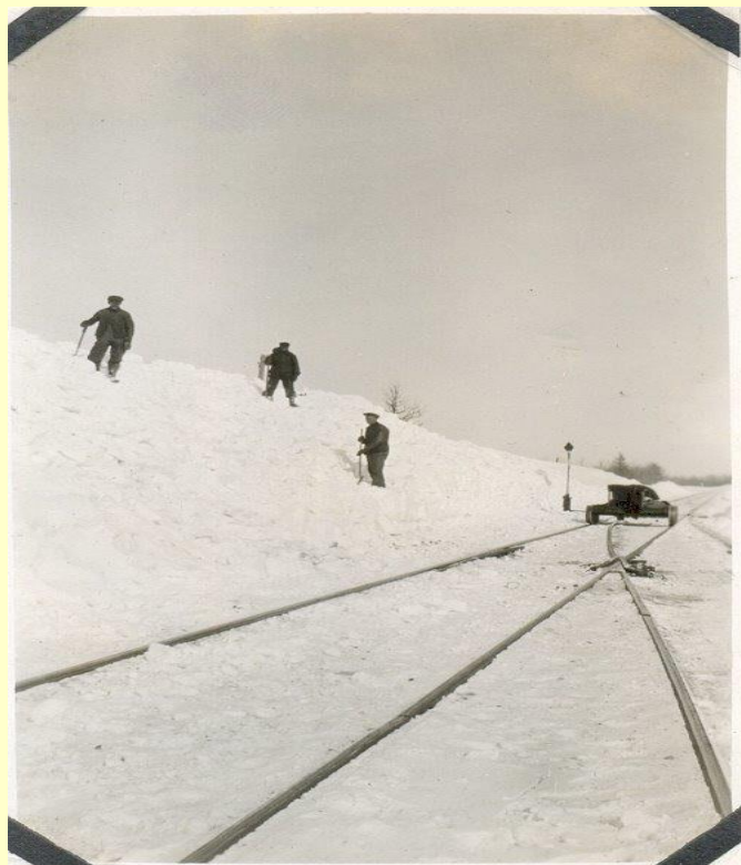
Men clearing the railroad tracks near Brandon after the Armistice Day storm in 1940.
