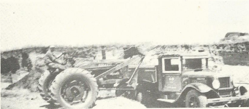
GRAVEL LOADING WITH a Farmall tractor and a B4 International truck, a 1934 model with a wooden cab.
