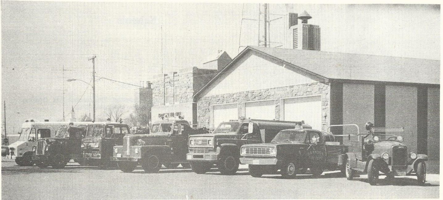
IN FRONT of the new fire barn: (Left to Right) fire equipment van, John Bean, Max Pumper, Pirsch No. 4, tanker,
