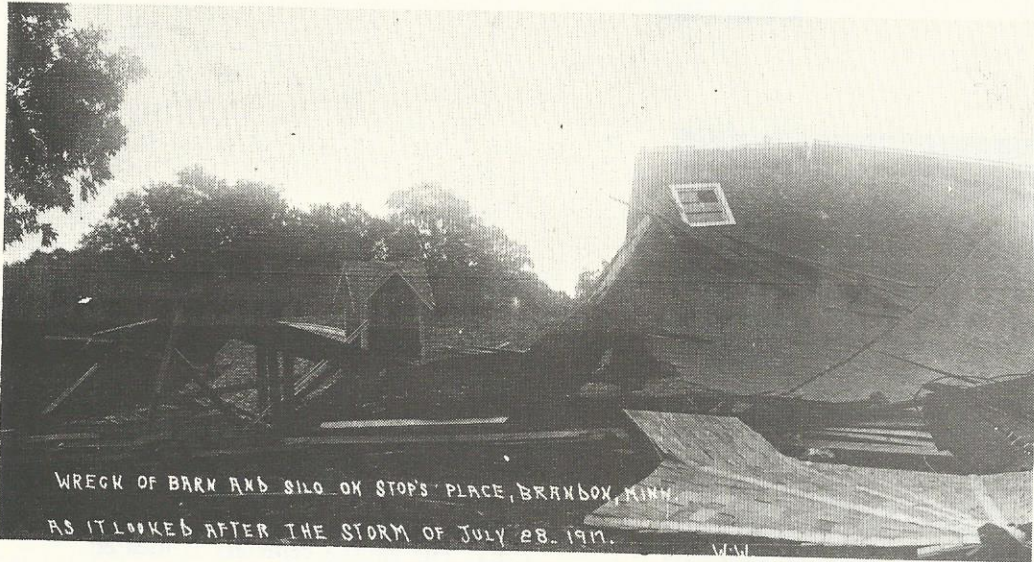
WRECK OF BARN and silo on Stop's farm as it looked after the storm of July 28, 1917.
