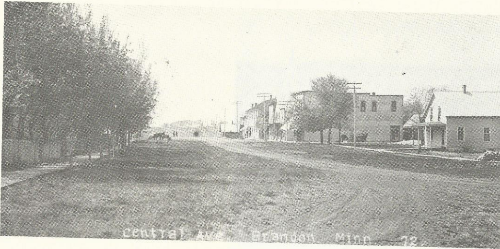
LOOKING SOUTH - early 1900 Central Avenue
