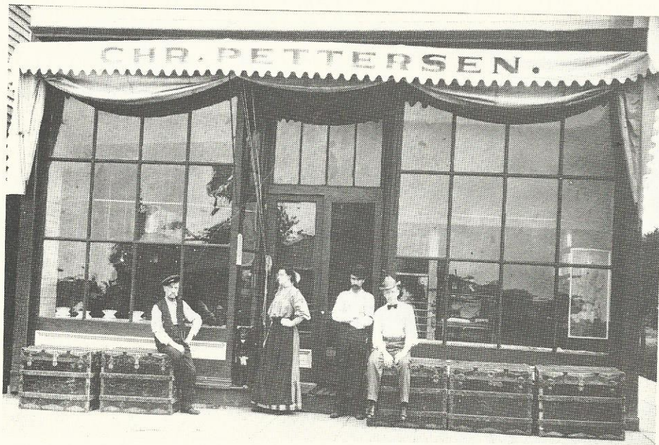
THE CORNER OF Front Street and Holmes Avenue. The laundromat is now on this site.
