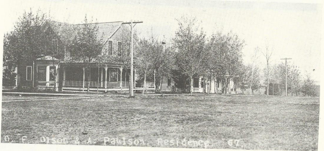
THE O.F. OLSON HOME was destroyed by fire, rebuilt by J.O. Renkes, and is now the home of Wm. Killmp.
