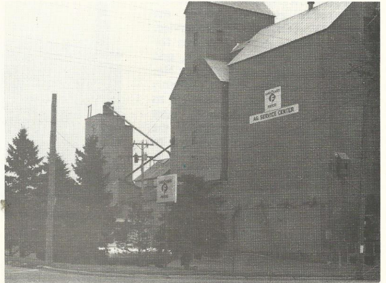
THE LAND O LAKES elevator as it appears today.
