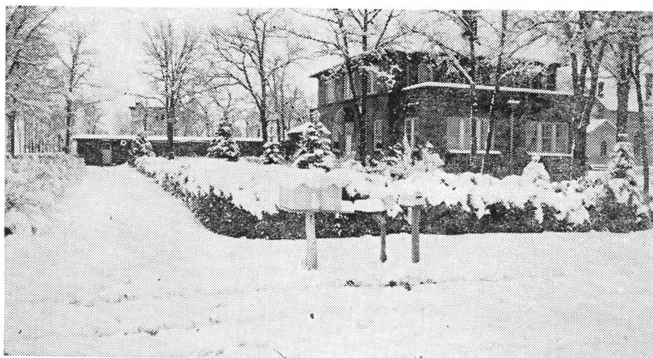
A view of the parish house with the entry to the basement church built by Father Siegler in 1923. The west end of the church. The picture is taken from the south.
